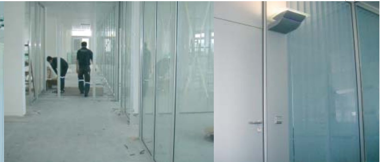
Top: the MAN offices during renovation
